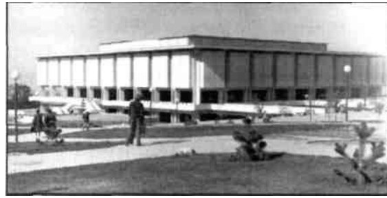
Marriott Library on the campus of the University of Utah at Salt Lake City, Utah.
